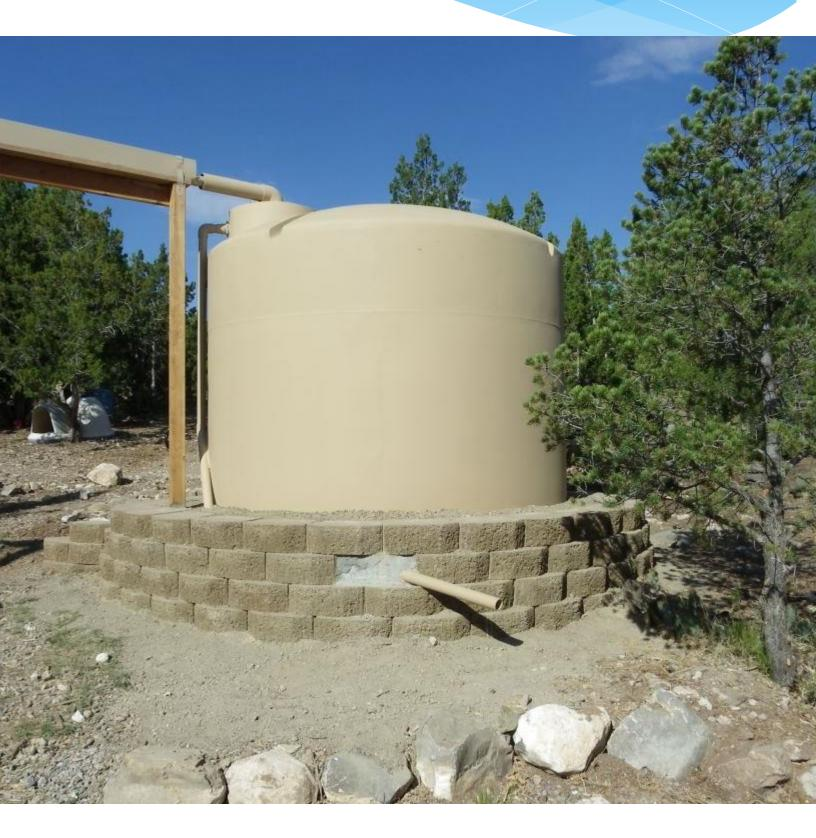
During a 1" rainfall – for every 1,000 sq. ft. of roof surface with a 90% roof efficiency, there is a potential to conserve 623 Gallons of Water!
